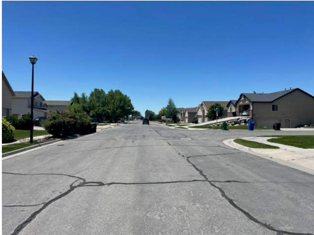
Looking westerly along 25 South near the west boundary of the subject.
